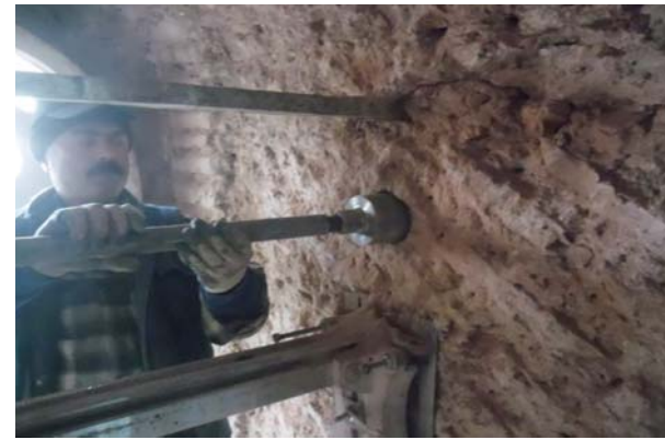
Picture 42. Beyazıt Mosque main dome tambour new reinforcement implementation detail (2013)
