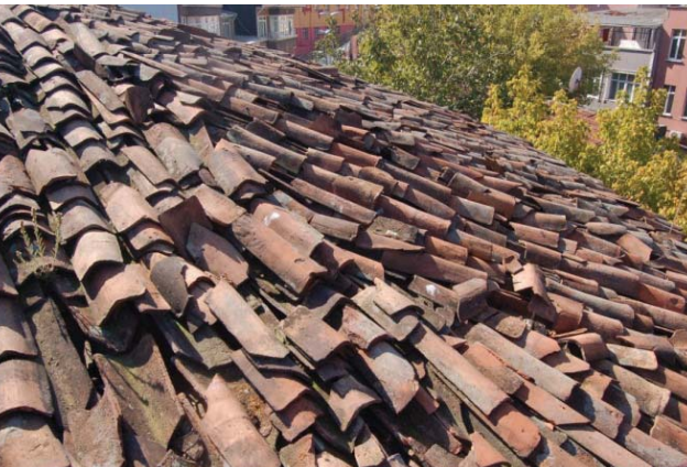
Picture 2. Pantiled roof (Before the restoration)
