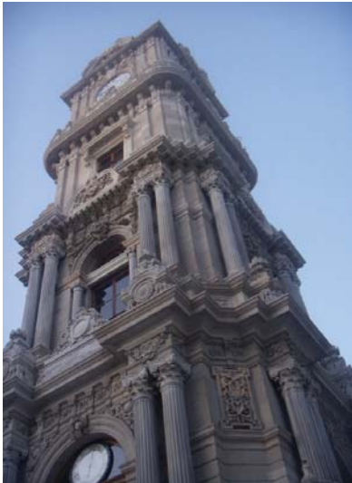
Picture 1. Tower overview after the restoration
