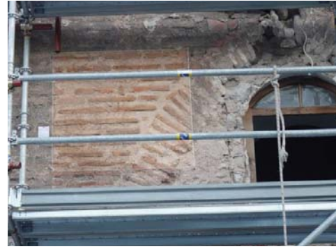
Picture 3. External – Cleaning sample – Picture by Leonardo s.r.l.
