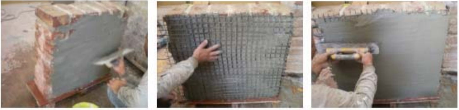
Picture 5. Retrofitting of the walls with TRM
