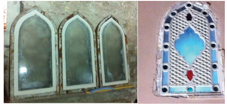
Picture 6. Renovated top windows (E. Sünnetçi, 2011)
