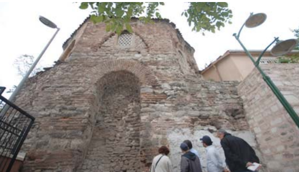
Picture 32. View of the east façade before the restoration
