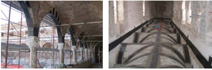
Picture 8. Strengthening technique: FRP strips system
