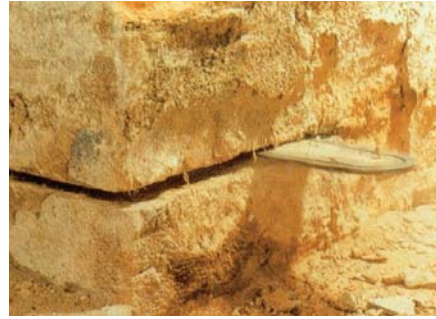
Picture 4. Mechanical cutting Resim 4. Mekanik kesim
