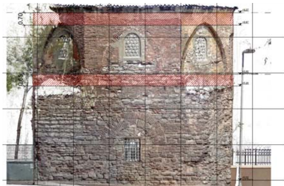
Picture 5. Strengthening project: steel strands confinement of masonry walls of Masjid
