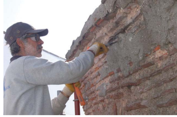
Picture 27. Scraping of the cement plaster
