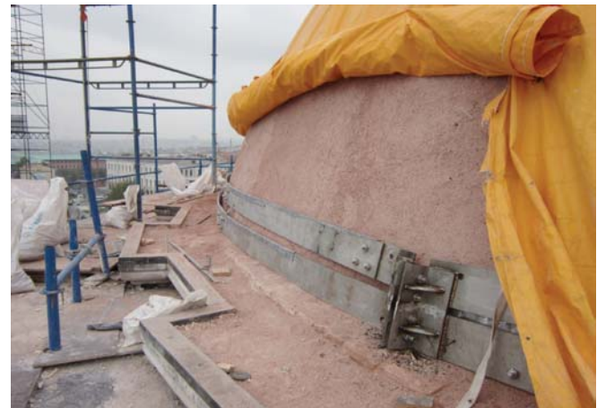
Picture 30. Beyazıt Mosque main dome tensile circle detail (2013)
