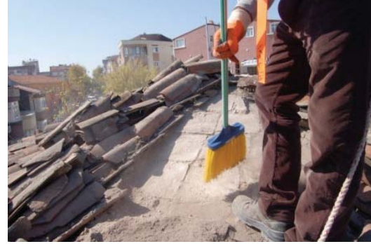
Picture 17. The tiles being removed and the soil being cleaned
