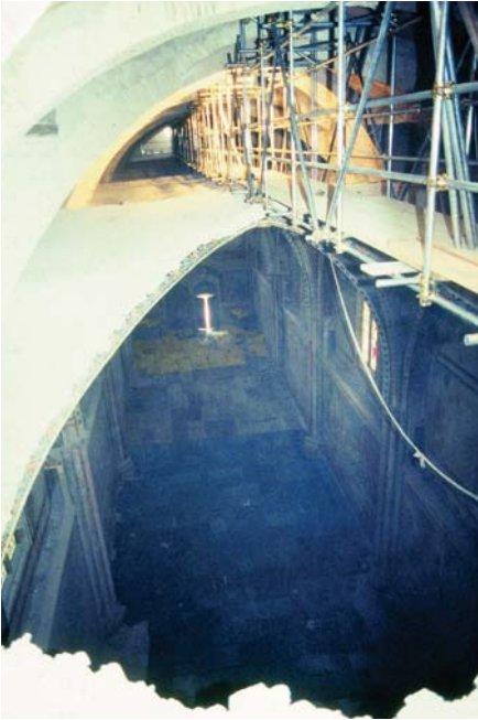
Picture 19. The Basilica of St. Francis in Assisi: The provisional "flying bridge" suspended to the roof
