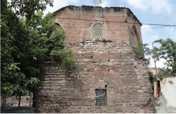
Picture 5. South façade view
