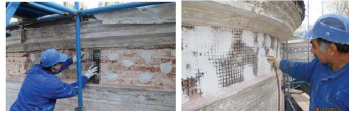
Picture 8. TRM applied zones and application steps
