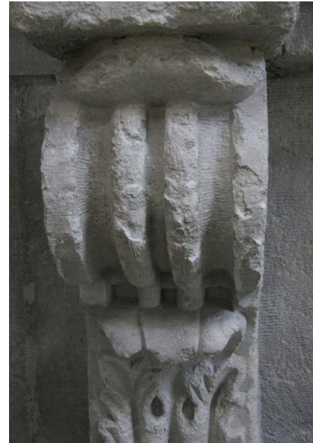
Picture 6. Restoration works (2008): final result after the surface consolidation and pointing
