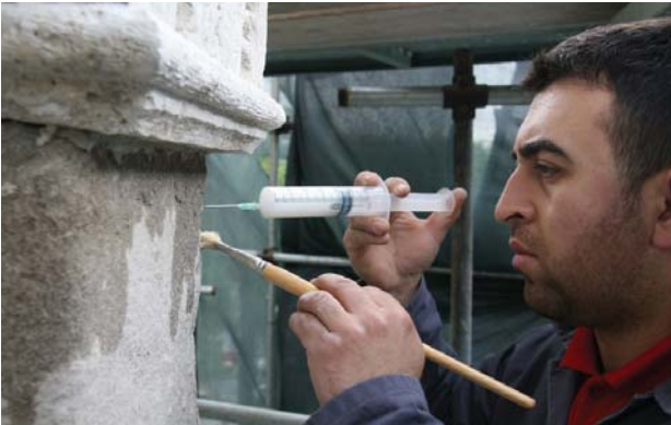
Picture 5. Restoration works (2008): on site pre-consolidation injection
