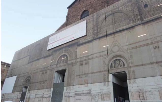
Picture 7. Scaffold canvas during façade restoration. St. Petronio Basilica, Bologna
