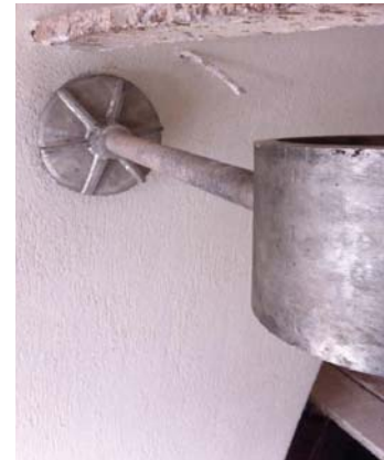
Picture 43. Beyazıt Mosque main dome tambour new reinforcement implementation detail (2013)
