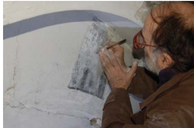
Picture 42. During the scraping
