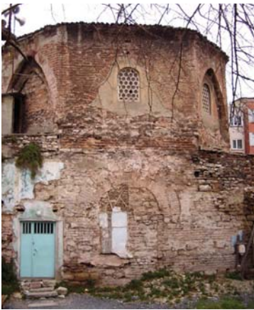
Picture 9. West façade of the Masjid. The original entrance which was blocked in two phases, can be seen in the centre of the façade. The photograph was taken in 2006 and after this date a platform was built on the yard and the level was raised. The beam gain which has the traces of a fire, can be seen on the left side of the façade.
