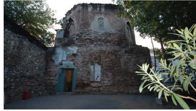
Picture 6. Forecourt (West) façade (on the left, the wall of the parking lot which is to be nationalized)
