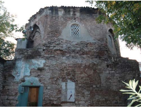
Picture 31. View of the west façade before the restoration
