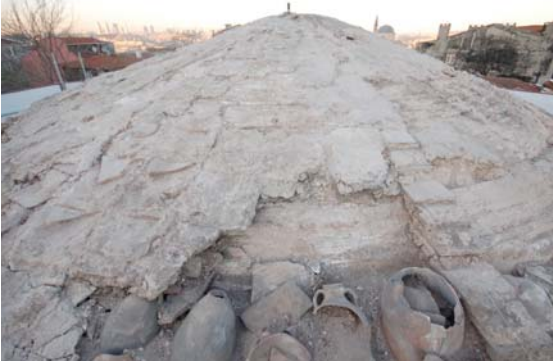
Picture 19. The view of the roof after the tiles have been removed and the soil has been cleaned
