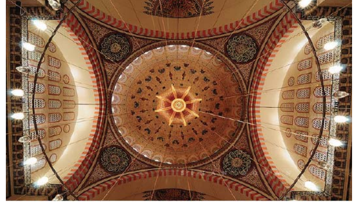
Picture 9. After restoration of main dome
