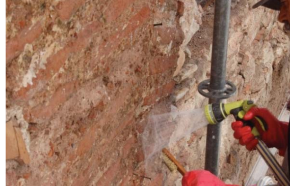
Picture 29. Cleaning the façade with water
