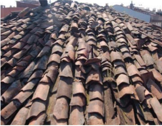
Picture 16. Tiled roof
