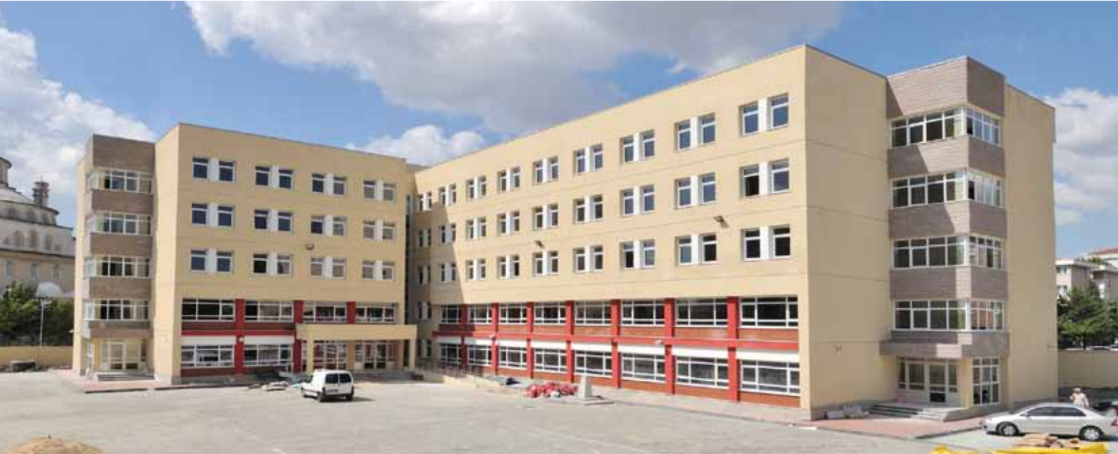
After Reconstruction, Kazım Karabekir Primary School, Bahçelievler
