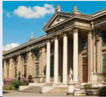
❖ Archeology Museum, seismic performance assessment completed and retrofitting operations in progress
