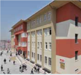
❖ Tuzla Peyami Safa Primary School, reconstructed
