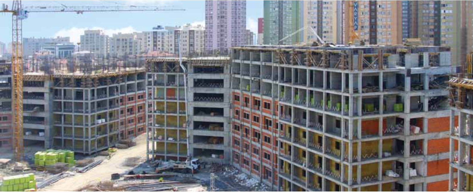
Atatürk Student Dormitory under Reconstruction, Zeytinburnu
