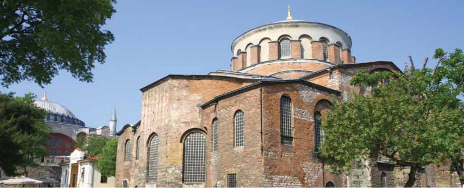
Hagia Irene, its Seismic Performance Assessed and Retrofitting Project Prepared
