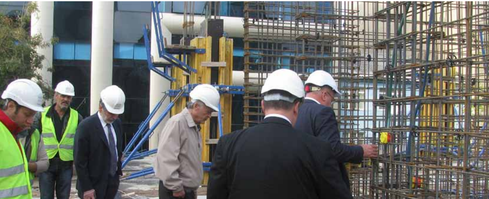
Examining of Reconstruction Works by the Project Technical Team
