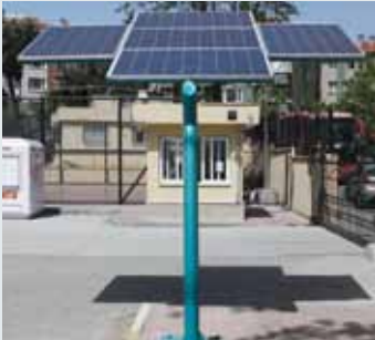
❖ Kazım Karabekir Primary/Secondary School, Bahçelievler, reconstructed, "Solar Tree"
