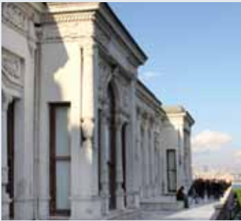
❖ Topkapı Palace, Mecidiye Mansion, retrofitting project completed
